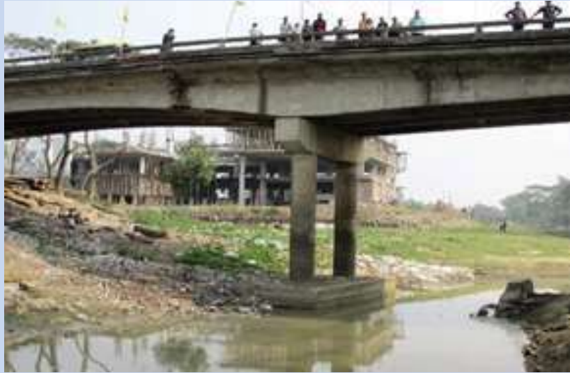
Figure-9: Low height Bridge.
