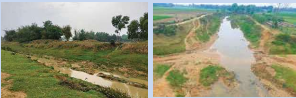
Figure-13: Due to BWDB Excavated soil the connection between river and canal has been blocked.
